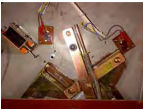
Locking Solenoid & Micro-switches-Detail
