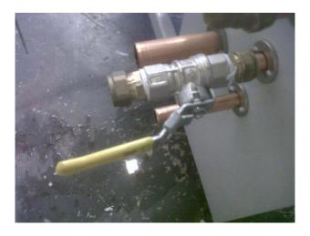
Allow the Steam Generator to release all of its pressure and fully drain the water. This should take approximately 10 minutes.
