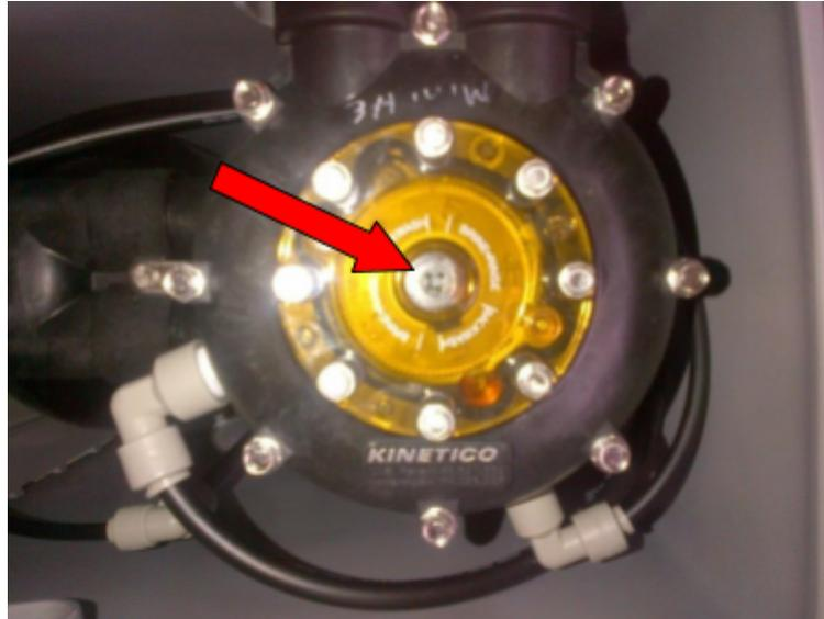
Using a Cross Head Screwdriver (recommended size PH2), push down firmly on the softener valve and slowly turn **CLOCKWISE** until the actuator has advanced the indicator **DOT** the 'BRINE' position. You should hear at least five clicks while turning the screw before the indicator **DOT** reaches the 'BRINE' position. At that point you will hear water flowing to the drain. This indicates that you have successfully initiated the start of the regeneration process.
