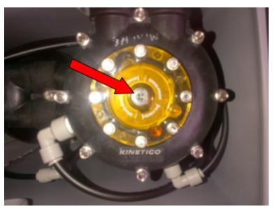
Using a Cross Head Screwdriver (recommended size PH2), push down firmly on the softener valve and slowly turn CLOCKWISE until the actuator has advanced the indicator DOT the 'BRINE' position. You should head at least five clicks while turning the screw before the indicator DOT reaches the 'BRINE' position. At that point you will hear water flowing to the drain. This indicates that you have successfully initiated the start of the regeneration process.
